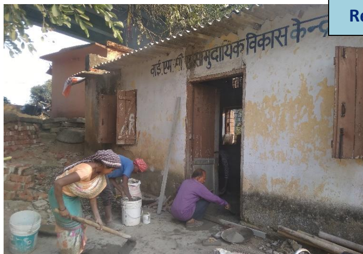
Preparing the walls for the new roof sheets after removal of old asbestos sheets.
