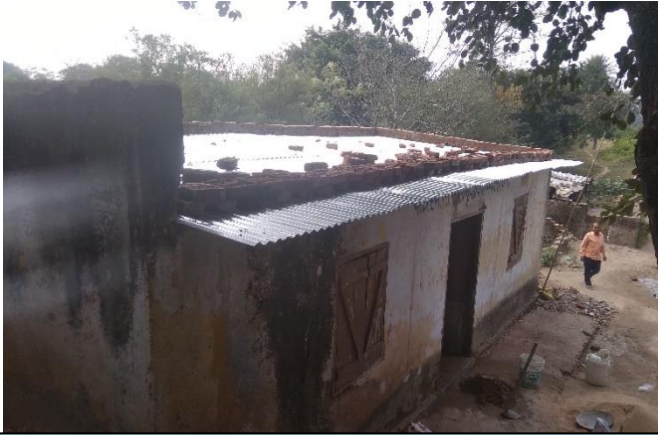
After installation of new steel roof sheets
