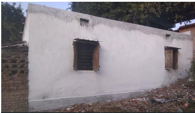
The backside of the building after repair, fresh plaster and first coat of paint.
