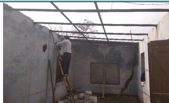
Preparing the walls for the new roof sheets after removal of old asbestos sheets.
